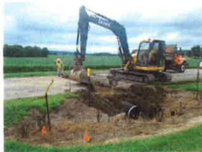
Culvert Replacement CR149 – Elyria Road
