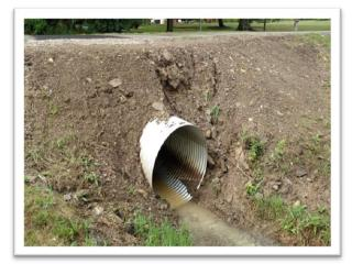
SUG 80-2.780 on Jericho Road in Sugar Creek Township. An existing 72" span x 44" rise metal pipe was replaced with 40' of 60" reinforced concrete pipe. Replacement work was completed by county forces. Local monies financed the project at a total cost of \$29,001.
