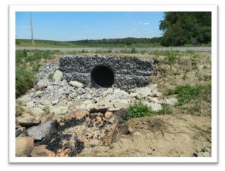
GRE 120-2.895 on Five Points Road in Green Township. An existing 48" metal pipe was replaced with 40' of 48" metal pipe. Replacement work was completed by county forces. Local monies financed the project at a total cost of \$7,048.
